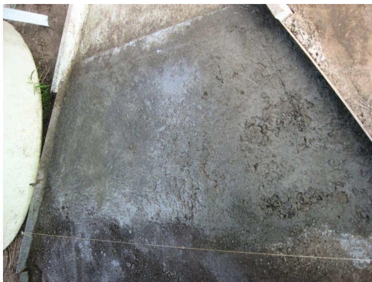
Figure 5.14 A thin strip of the entrance covered with sprinkles of Portland concrete cement.
